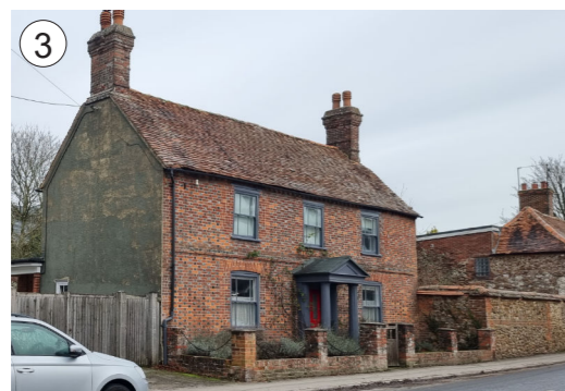
Grade II - 22 Oxford Street - C18, 2 storeys house built of brick with grey headers and red stretchers. It has a 1st floor string course, dentil work on the eaves. Clay tile roof with flanking chimneys. Vertical sliding sash windows, glazing altered, under brick arches wider than present openings.
