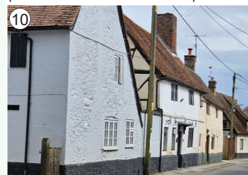
10 Newbury Street looking southeast, highlighting the row of listed terraced cottages.
