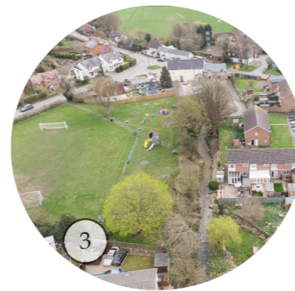
3 The play area at Mill Lane bounds the river on one side with late 20th Century dwellings at Tubbs Farm Close and Aintree on the other. Here the banks of the river appear to be eroding.
