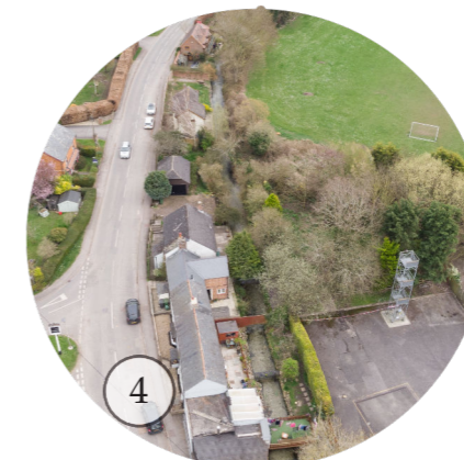
4 At the Fire Station and behind properties on Newbury Street, there is little space between buildings and the river. In some instances properties have bridged the river to allow for greater amenity space.
