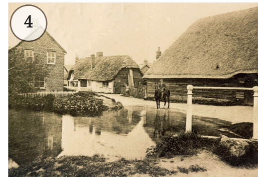
Bottom Bridge shown in 1910 looking towards the Barn to the south of Stable House and The Cottage - Newbury Road
