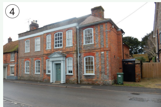
Grade II - 21 Newbury Street - C18. 2 storey house with an unsymmetrical facade - built of red / vitreous brick on a red brick plinth. Brick quoins and framing around openings. Brick banding at 1st floor. Brick parapet with stone coping. Clay tile roof with flanking chimneys. Vertical sliding sash windows.
