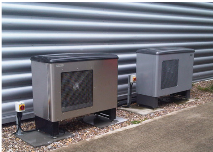
Figure 3. Air Source Heat Pumps
