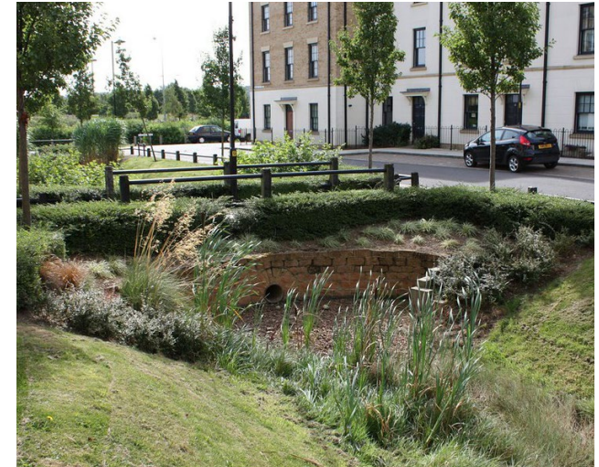
Figure 116: Example of swales check dam integrated with a crossing point, somewhere in UK.
