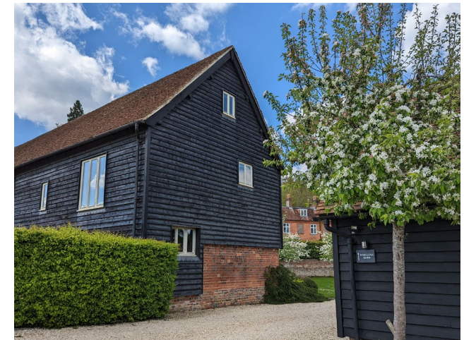
Figure 71: Local example of a barn that was converted into residential retaining the existing characteristics and materials of its former use.
