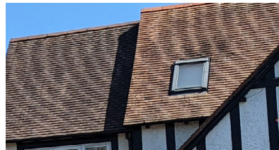
Red clay tiles on a gabled roof
