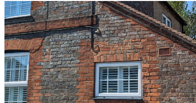
Variations of brick colour on facade
