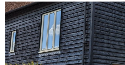
Modern windows on a converted barn
