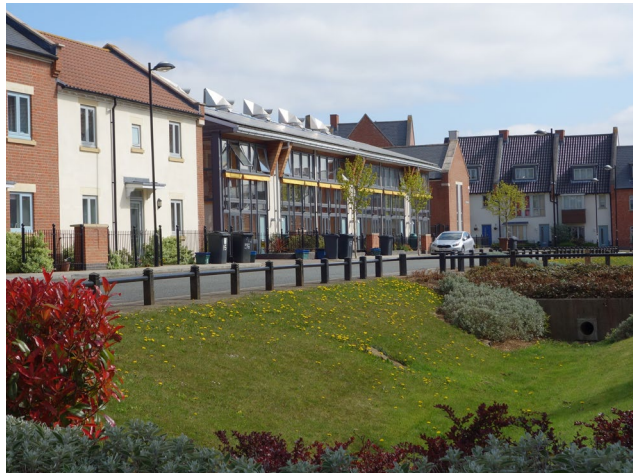
Figure 109: An example of a SuDS corridor - Upton Urban Extension, Northampton.
