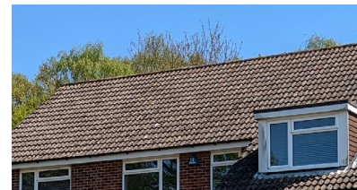
Red clay tiles on a gabled roof with dormer window
