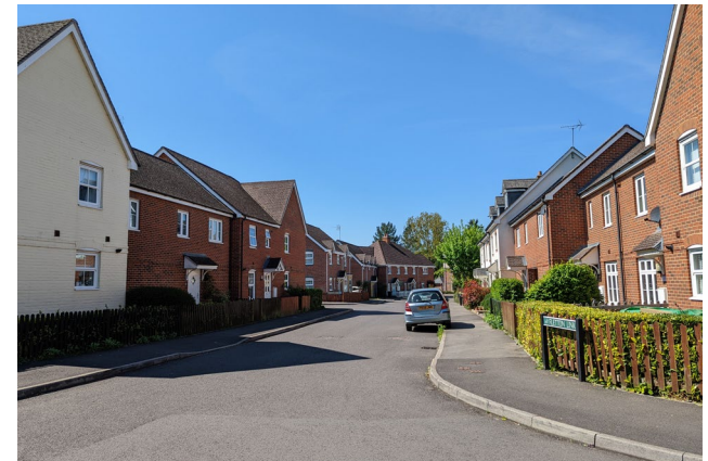
Figure 03: Fletton Link - a residential cul-de-sac characterised by pavements on both sides of the road and properties with smaller setback from the road.
