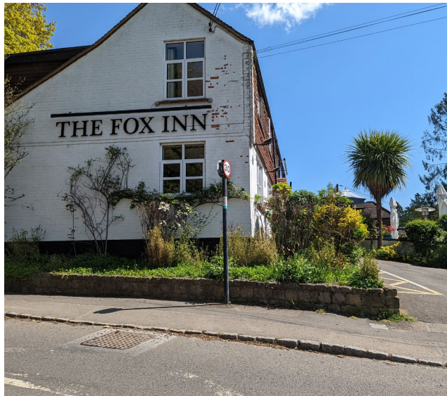
Figure 10: The Fox Inn pub is located in the corner of the junction of spine road (B4009) and Yattendon Road and it acts as a landmark for the village.
