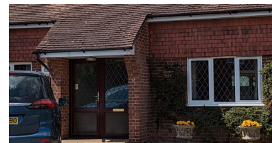
Porch under a catslide roof
