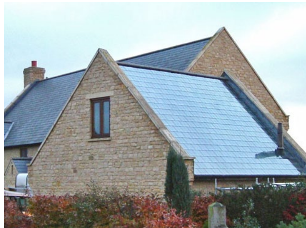
Figure 132: Positive example of implementing solar panels from the design stage.
