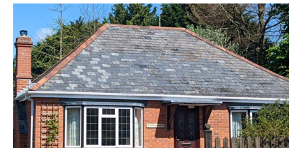
Grey slate tiles on a hipped roof
