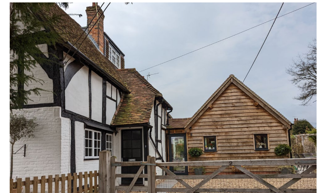
Figure 72: Positive example of a side extension that respects the existing building in terms of scale and building materials. In particular, the use of weatherboarding positively reflects back to the typical appearance of barns and outbuildings, elsewhere in UK.
