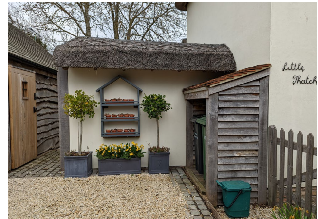
Figure 106: Local example where the bins are stored under the shed, whilst the side wall is decorated with flowers and plants to improve the environment. This arrangement combined with the particular permeable paving contributes to the rural feel of the village.
