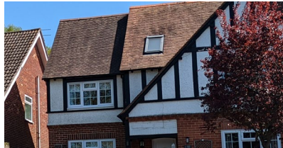
Timber frame with white render infills
