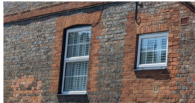
Sashed window framed with red brick
