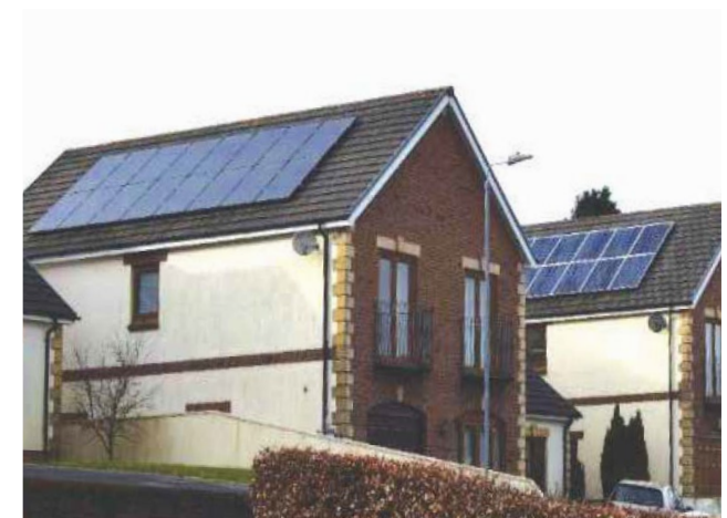
Figure 133: Positive example of implementing solar panels from the design stage.
