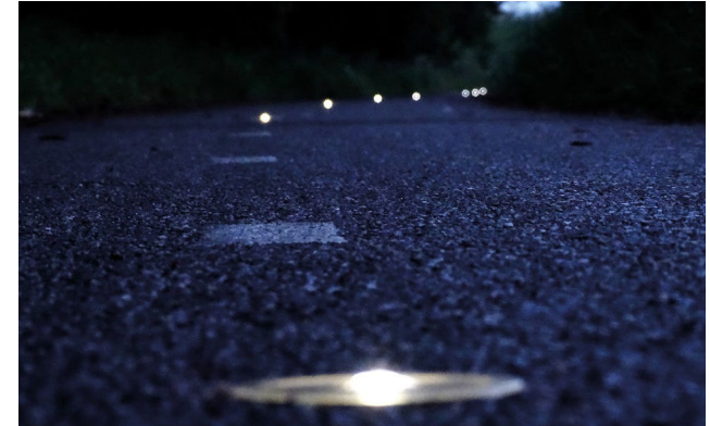
Figure 90: Example of a foot/cycle path which is lit by solar cat's-eye providing some light for pedestrian and cyclists without creating any disturbance to the nearby properties or unacceptable levels of light pollution.
