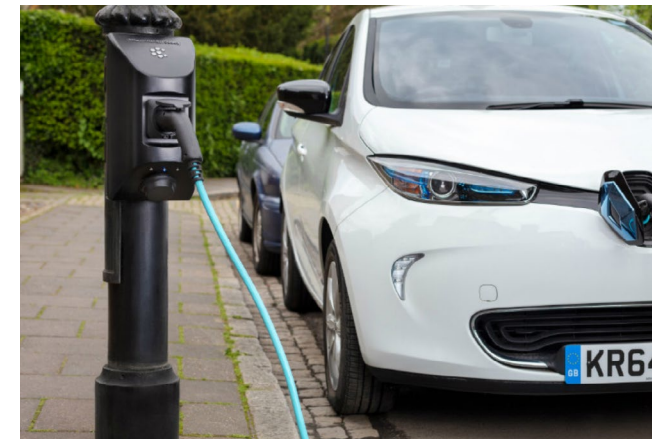
Figure 96: Example of on-street electric vehicle charging points.
