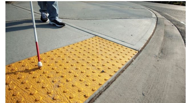
Figure 57: Example of tactile paving to facilitate movement for people with visual impairment.
