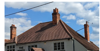
Hipped roof with red brick chimneys
