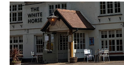
Gabled porch with wooden details appropriate for a commercial building
