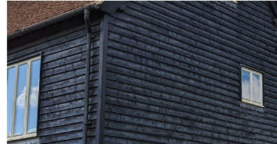
Horizontal dark weatherboarding
