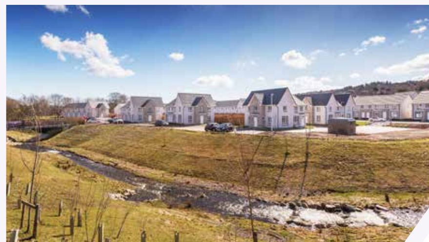
Views across the development and the 'daylighted' Bucks Burn which now provides a focus for the development and greater wildlife opportunities.
