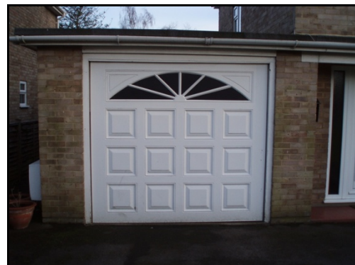
Garage attached to dwelling
