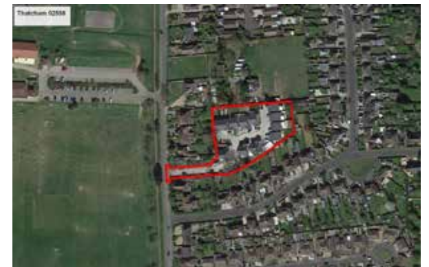
Figure 12: Infill housing on site with poorer access, Thatcham, 29dph
