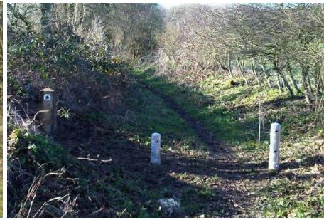
Council installed carriage gap
