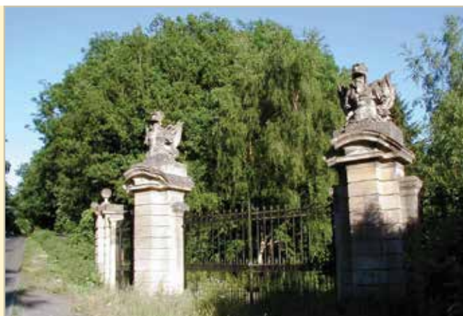
Speen: Benham Valence gate piers
