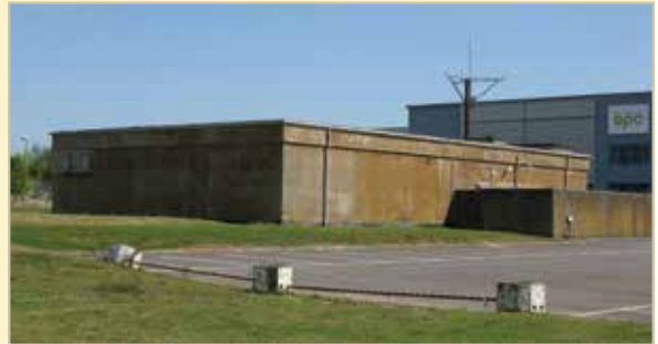
Greenham: Grade II listed Combat Support Building 273
