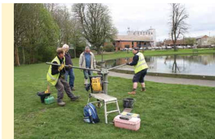
Newbury: Coring in Victoria Park
