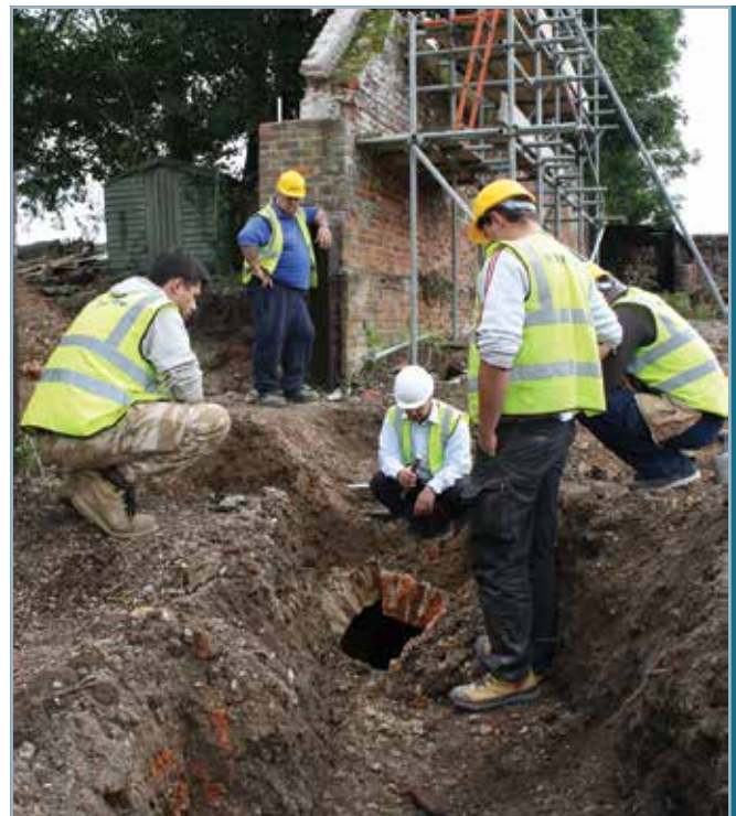
Hamstead Marshall: The discovery of the brick tunnel
