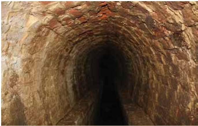
Hamstead Marshall: A view down the brick tunnel
