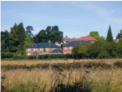
Infill development clearly visible from Moor Lane
