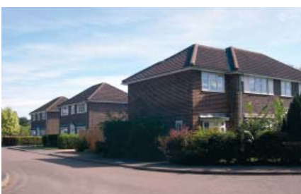
1970s cul de sac development characteristic of the infill on the northern side of Speen Lane
