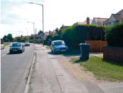
Deteriorated quality of public realm in places along Bath Road
