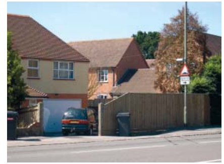
Example of erosion of mature landscaping and hedgerows, replaced with fencing and parking
