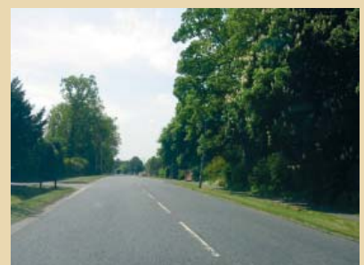
Maintain grass verges and mature landscaping along length of the road
