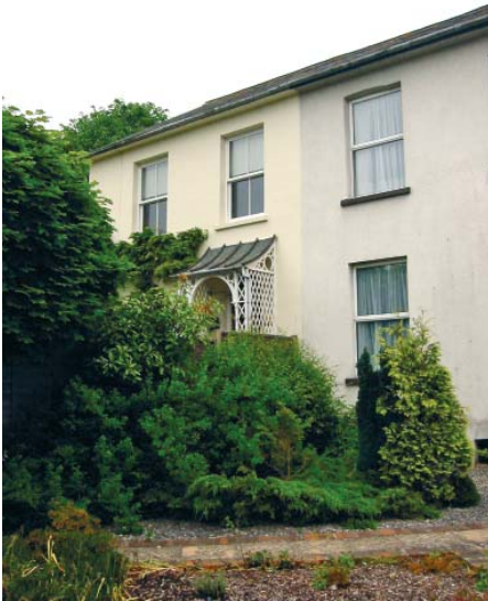
Victorian terraces with mature landscaping close to Gwyn Close
