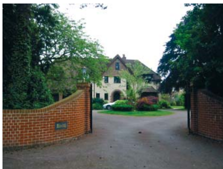
Key development sites such as the former hospital site will be brought forward in the near future and should be seen as an opportunity to enhance the character of the corridor
