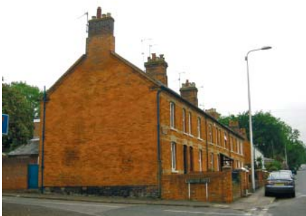
Victorian terrace along Andover Road
