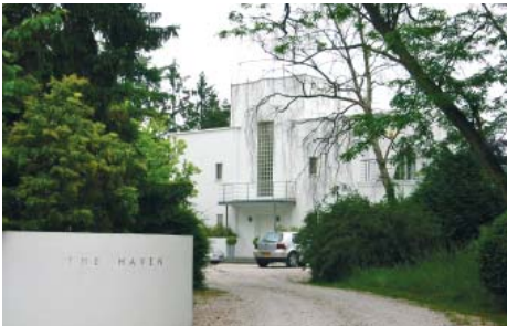
The Haven is a fine example of a large dwelling in the Internationale Moderne style and is one of many large properties located at Tydehams and Woodridge
